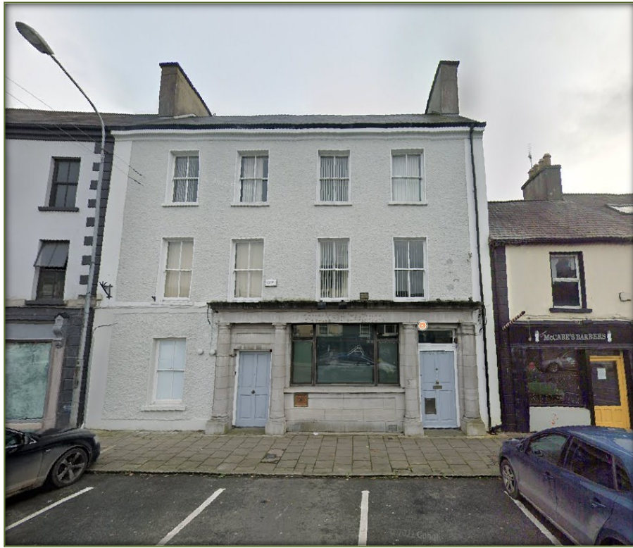
Figure 5a – Existing Front of Building (© Google)
