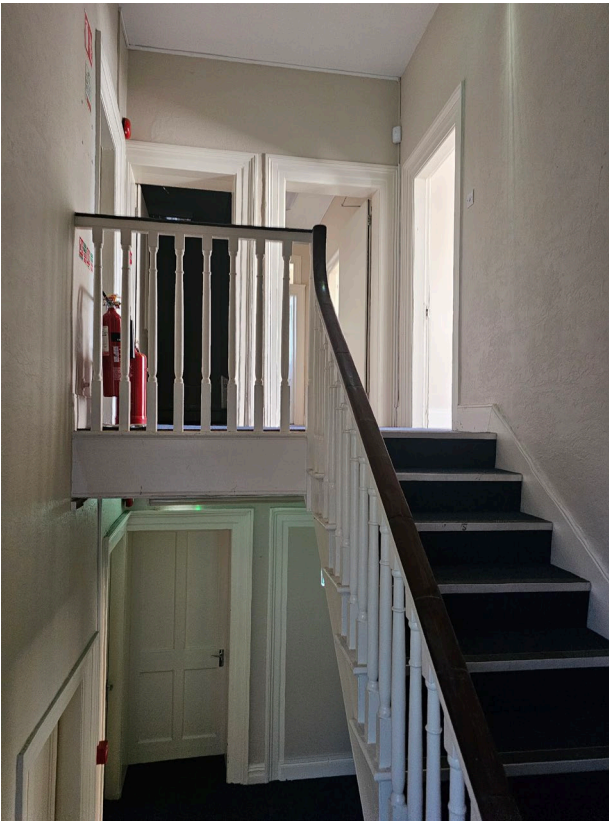
Fig. 19 – Internal Stairs to Second Floor
