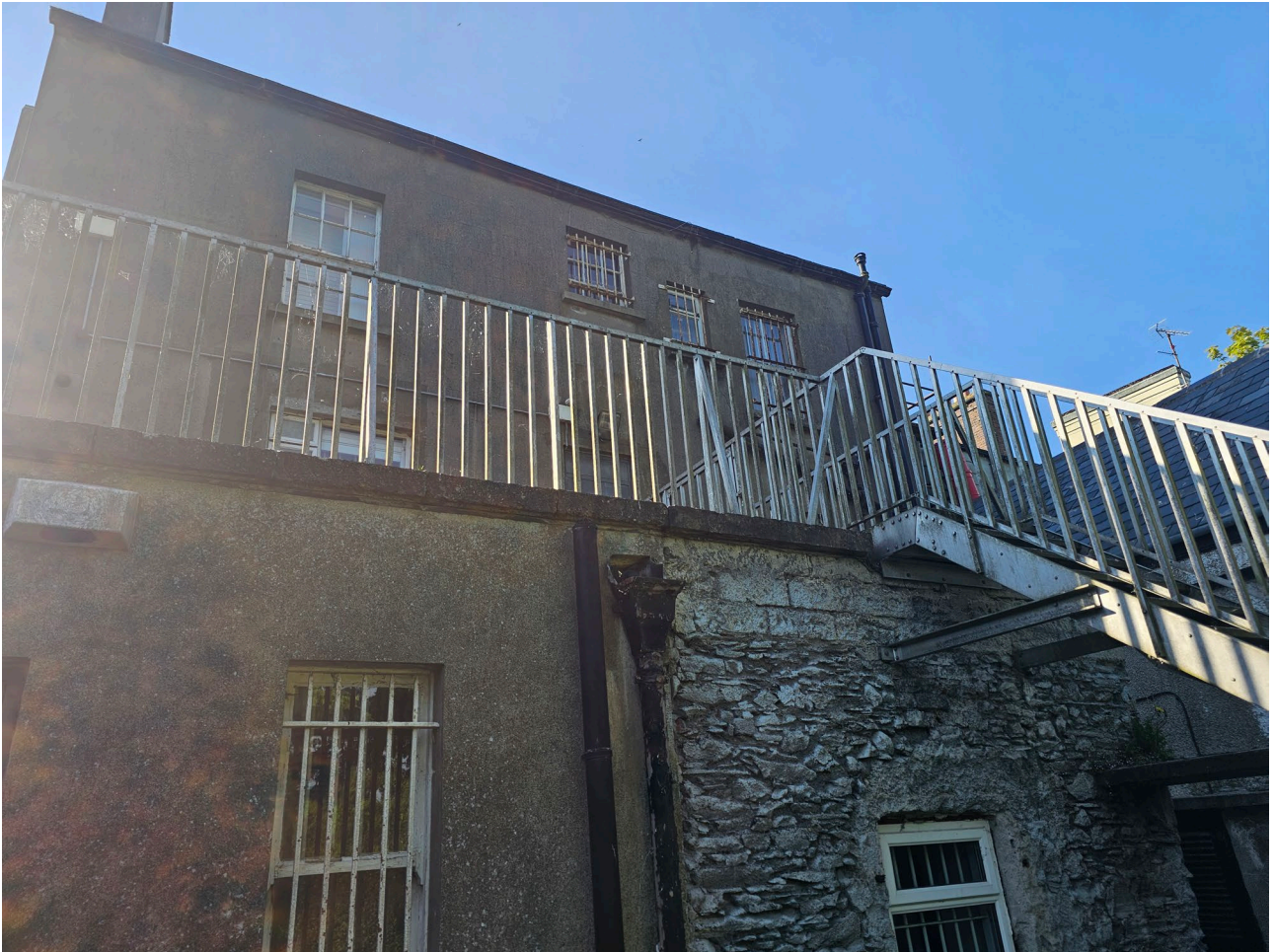
Fig. 2 - Rear Elevation of Building
