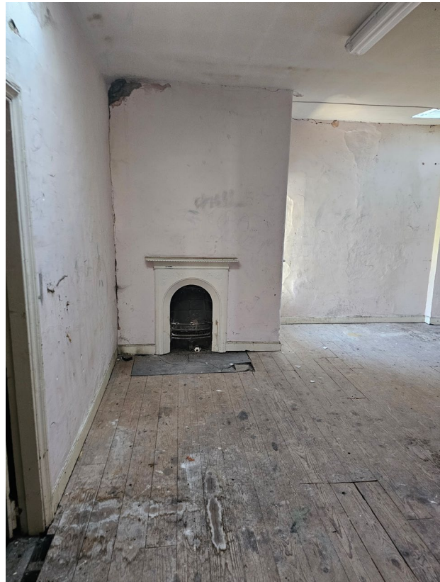
Fig.20 – Interior View of Third Floor
