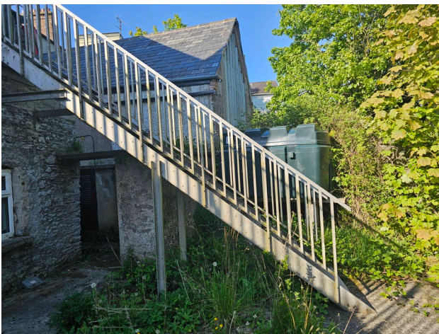
Fig. 4 – View of External Stairs
