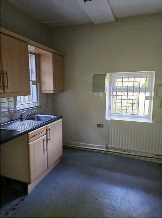
Fig. 9 – Ground Floor Interior – Existing Kitchenette to rear
