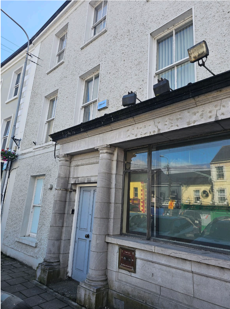
Fig. 1 - Front Elevation of Building
