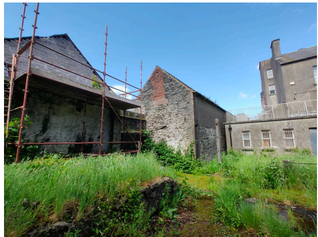
Fig. 5 – View of Adjacent Buildings
