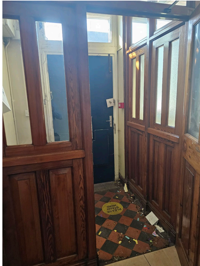
Fig. 6 – Ground Floor Entrance to Bank
